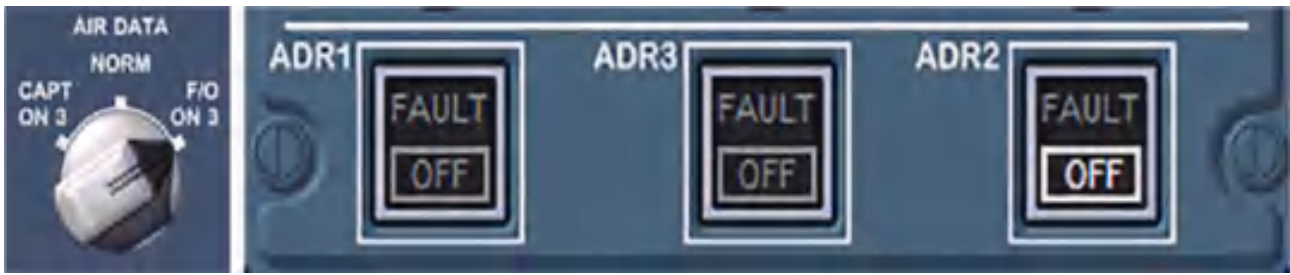
Figure 1. Application of MEL 30/31/01B for First Officer's Probe Heat Computer (PHC) inoperative. Instructions are to select the AIR DATA to [F/O ON 3] and set the ADR2 pushbutton switch to OFF prior to entering icing conditions.
